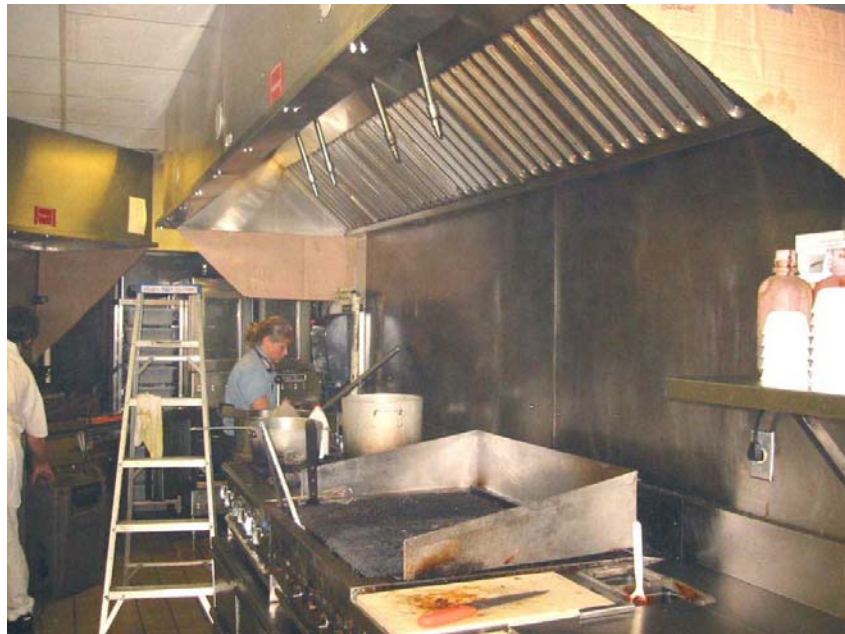
Figure 5. Hood 1 – cardboard mock-up of partial end panels.
