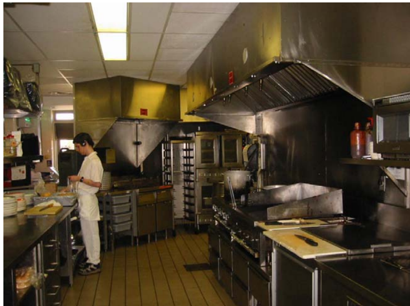
Figure 6. Stainless steel panels installed.
