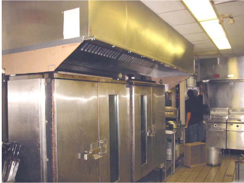
Figure 7. Hood 2 – cardboard mock-up of partial end panels.
