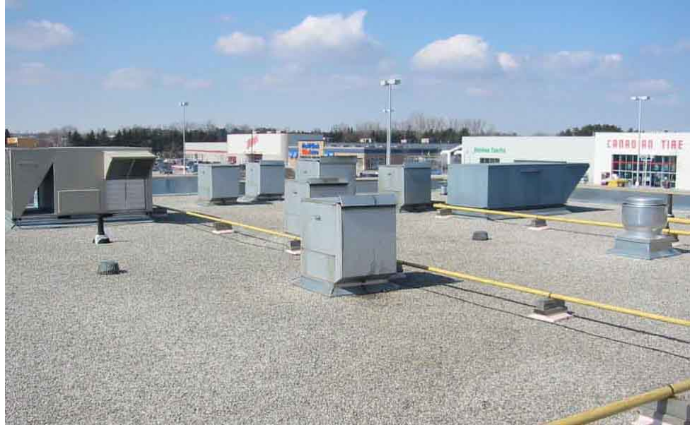
Figure 3. Rooftop perspective (showing 7 exhaust fans & MUA unit).
