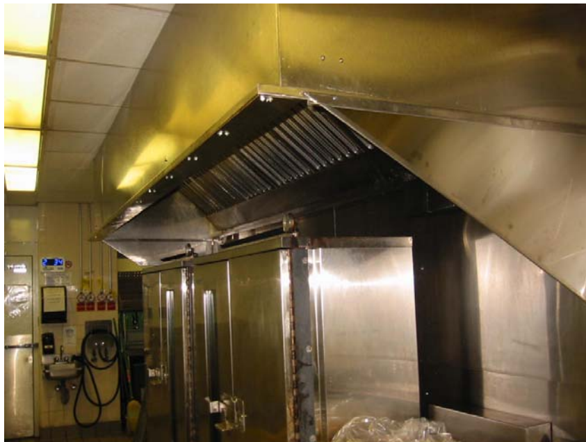
Figure 8. Hood 2 – stainless panels installed.
