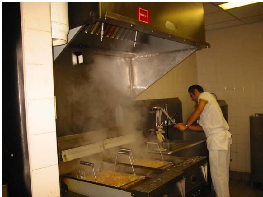
Figure 10. Fryer hood with end panels and complete capture.
