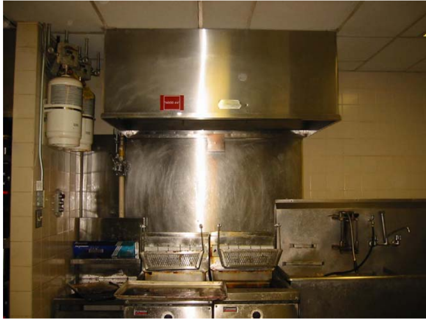
Figure 9. Fryer hood with open ends (and poor performance).
